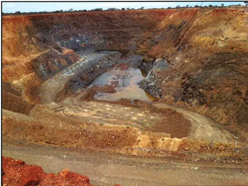
Plate 1. Butterfly Pit following the mining campaign of 2012, looking southeast after a recent rainstorm . The orebody continues to depth dipping toward the left of the photo (east-northeast).
