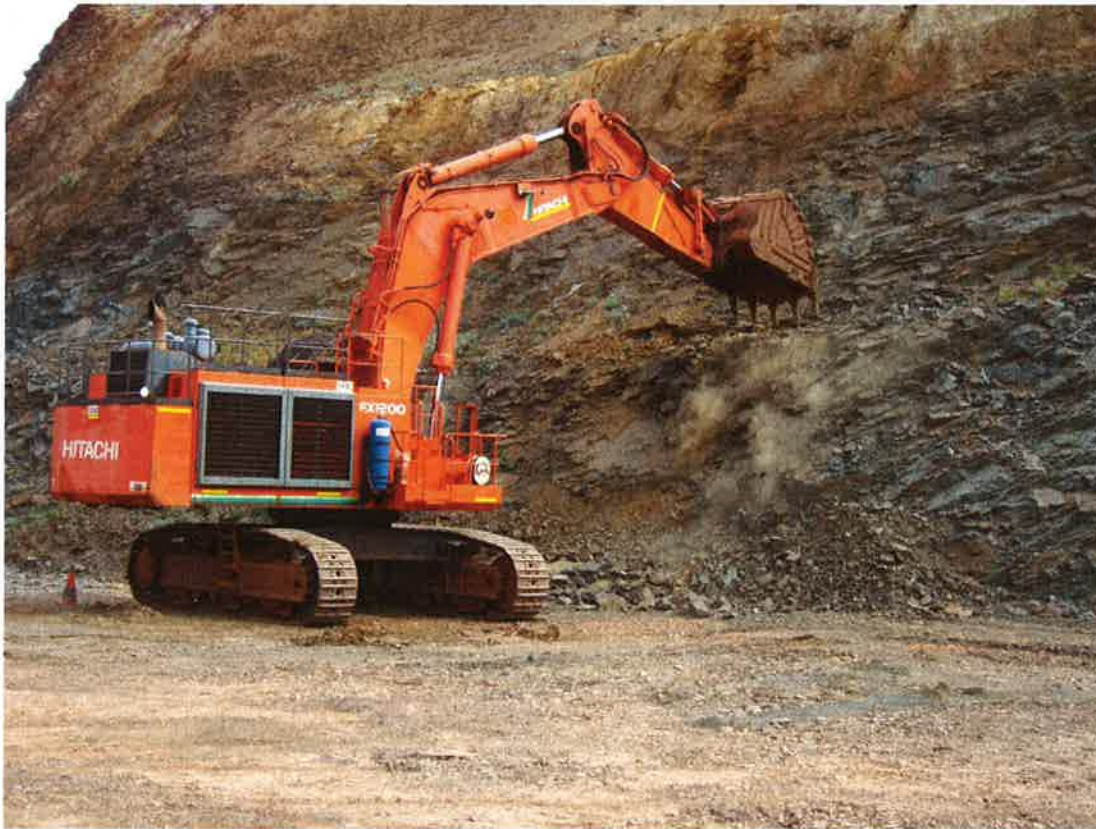
Photo 1. Excavator cleaning off berms and cutting batters prior to blast drilling.
