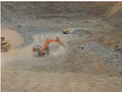
EX1200 pulling the final waste off the high grade ore under the supervision of geologists.
