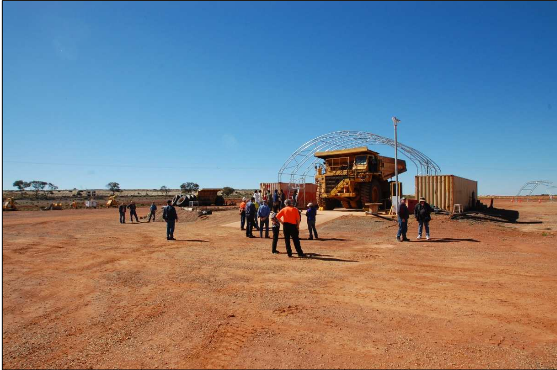
Photo 2. New maintenance shelter being installed for working on the mining fleet.
