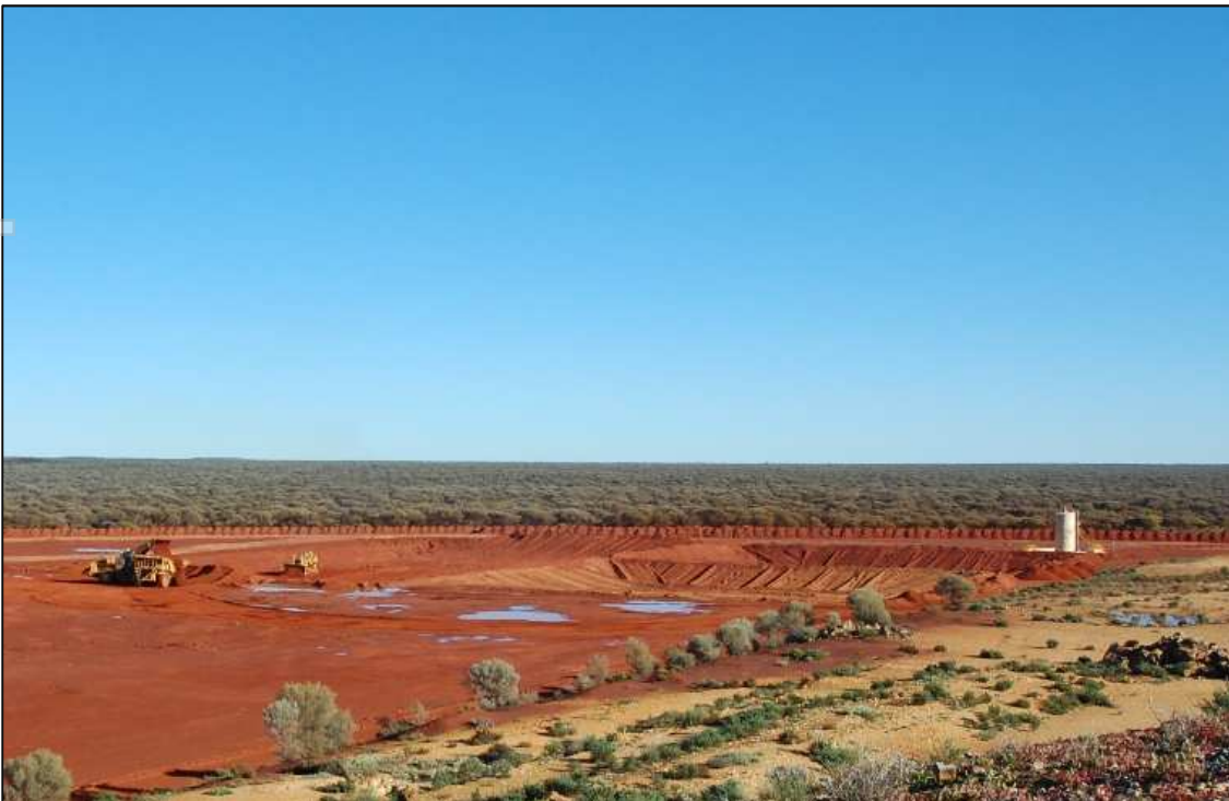
Photo 3. The Komatsu WA800-2, CAT D11N and one of the CAT 777Bs working in the stormwater pond with the pregnant and barren solution ponds and cyanide storage tank to the right.
